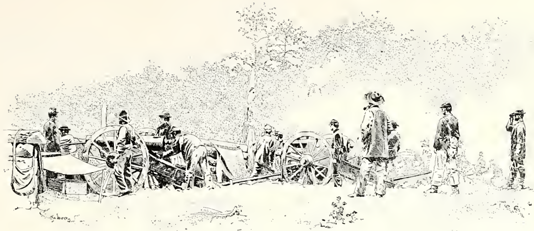
UNION BATTERY NEAR DUNN'S HOUSE, PETERSBURG. FROM A WAR-TIME PHOTOGRAPH.
